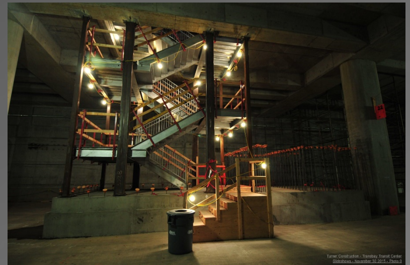
Below Right: Stair installation between Train Level and Lower Concourse.
