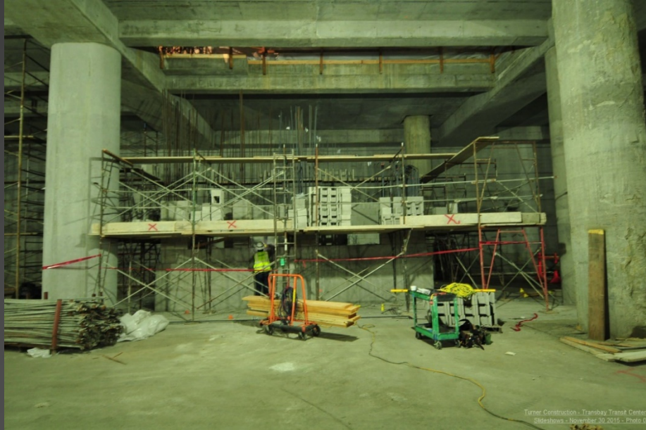
Above: CMU work at Train Level.
