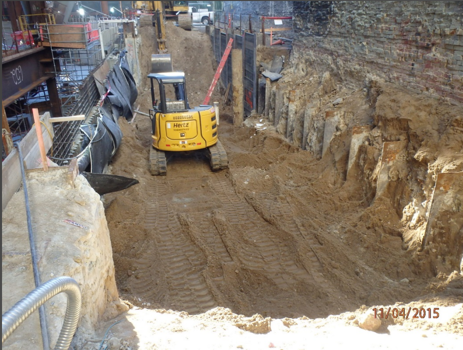
Above: Civil work at west end of project, preparation for Stair 201.
