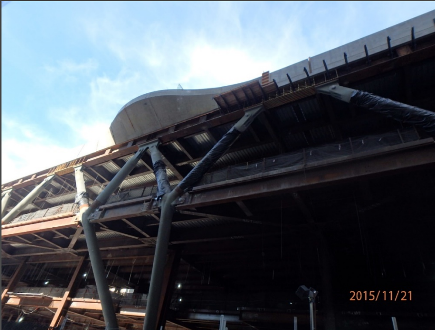
Above: Exterior view of first scallop wall completed.
