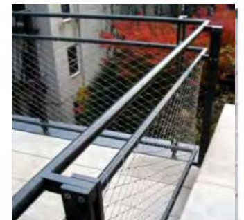
06 Stainless Steel Cable Mesh Gaurdrail
