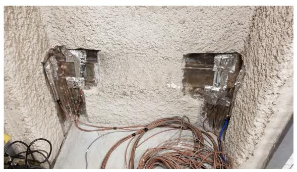
Building monitoring system has been installed on bus deck and locations below the bus deck
