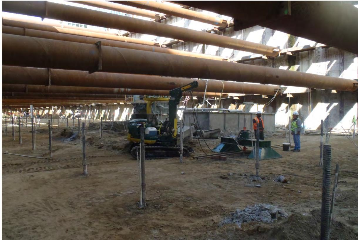
Micropile Pull Test Underway
