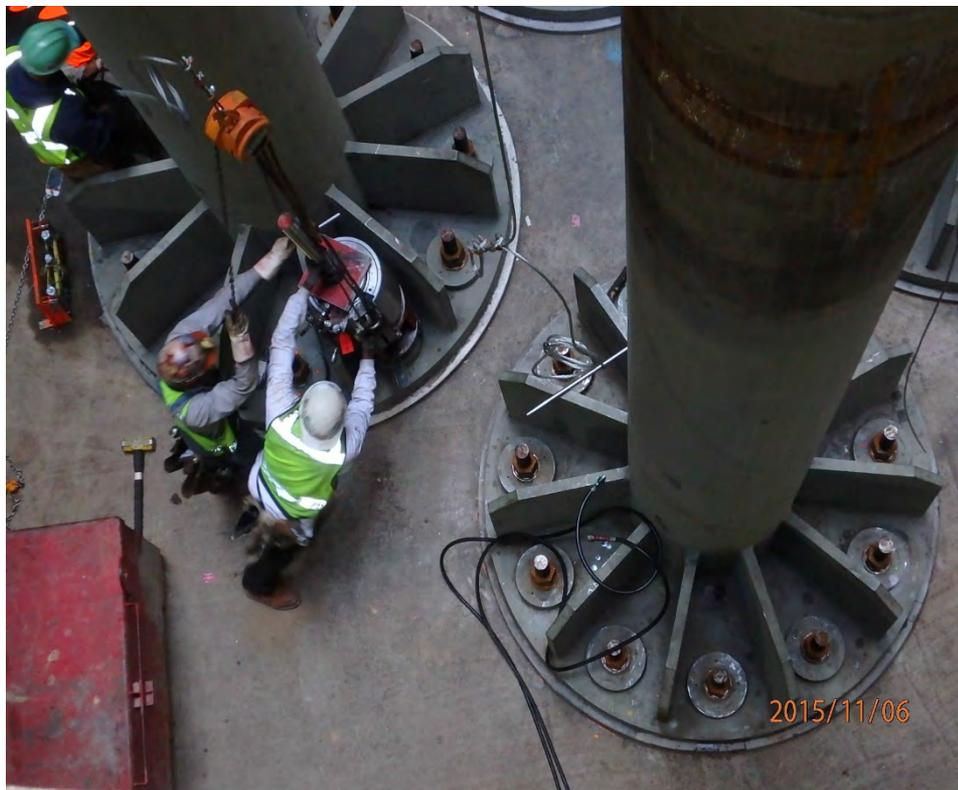
Bolt tensioning underway at Light Column
