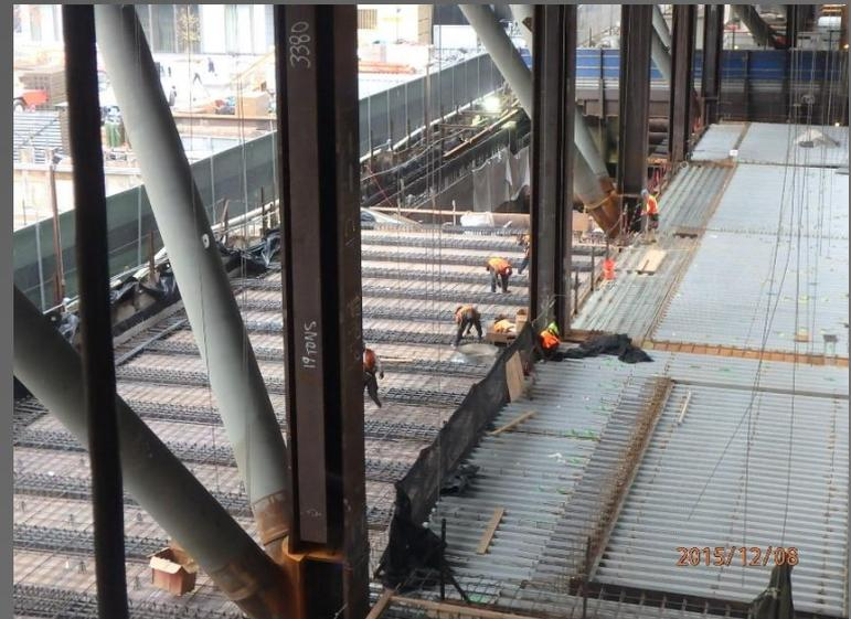
Above: Steel erection complete and trestle removal near completion.
