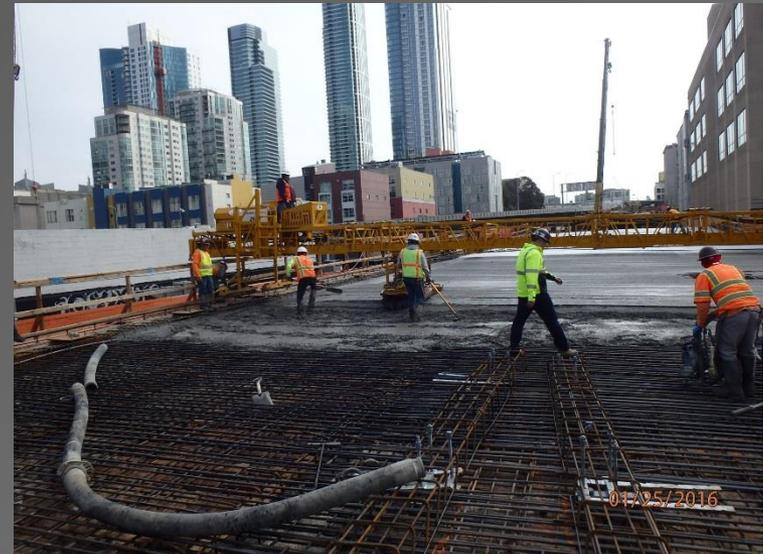
Below Right: Concrete placement at Tehama Street viaduct deck.
