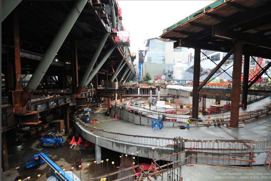
Above: Vehicle and bike ramp in progress at west end of project. Bus ramp falsework above ramps. Structural steel welding in progress.
