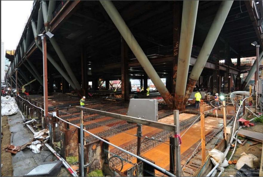
Above: Northwest corner eyebrow falsework, formwork and rebar in progress.
