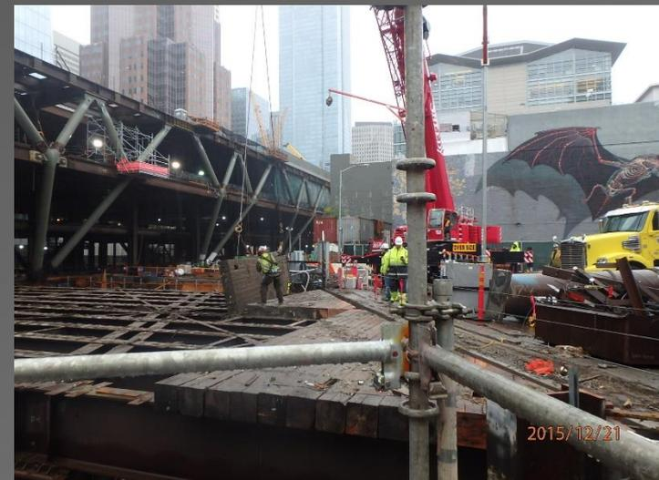
Above: Structural steel erection completion at the west end.
