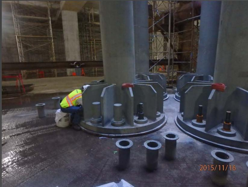
Above: Covering light column bolts after final testing.
