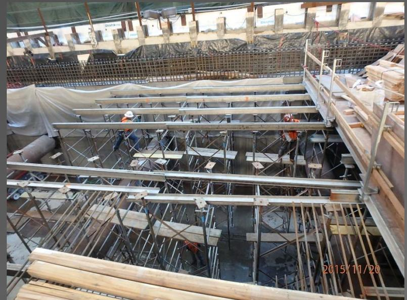
Above Right: Ongoing "eyebrow" formwork installation.
