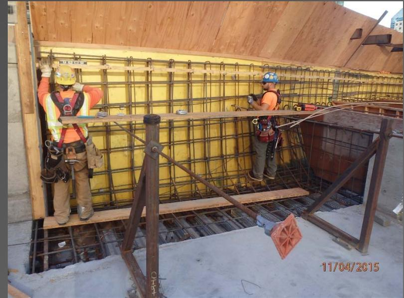
Above Right: Scallop wall formwork and reinforcing steel.
