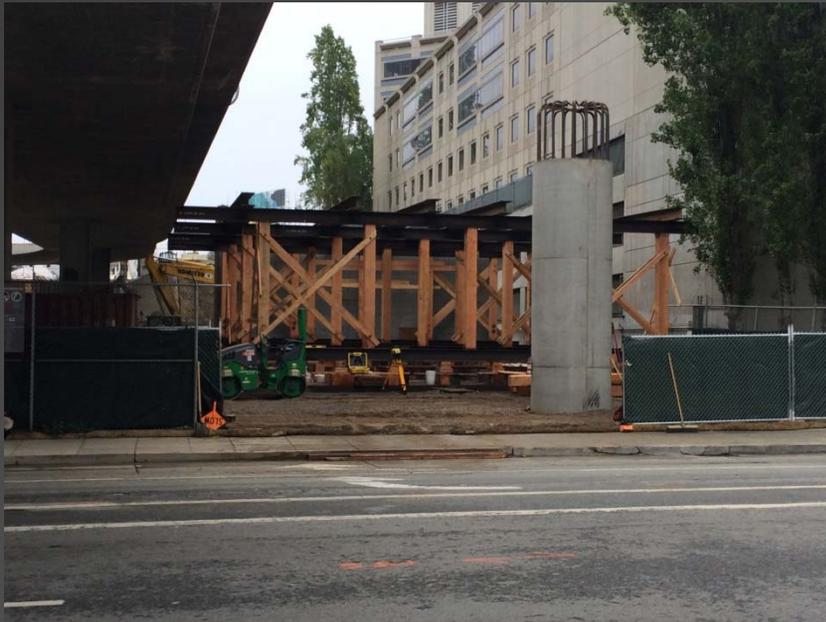
Above Left and Right: Falsework erection in progress, southside of Folsom Street.
