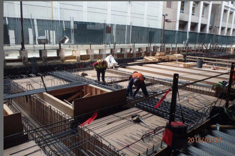
Below Right: Formwork for Train Box lid (eyebrow) concrete placement.
