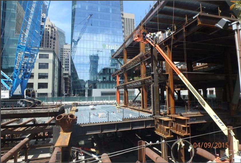
Above Left : Structural steel erection at gridline 9 proceeding west.
