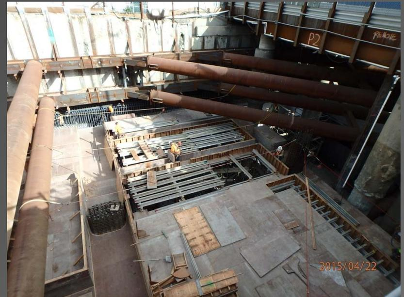
Above Right: On going installation of Lower Concourse formwork.
