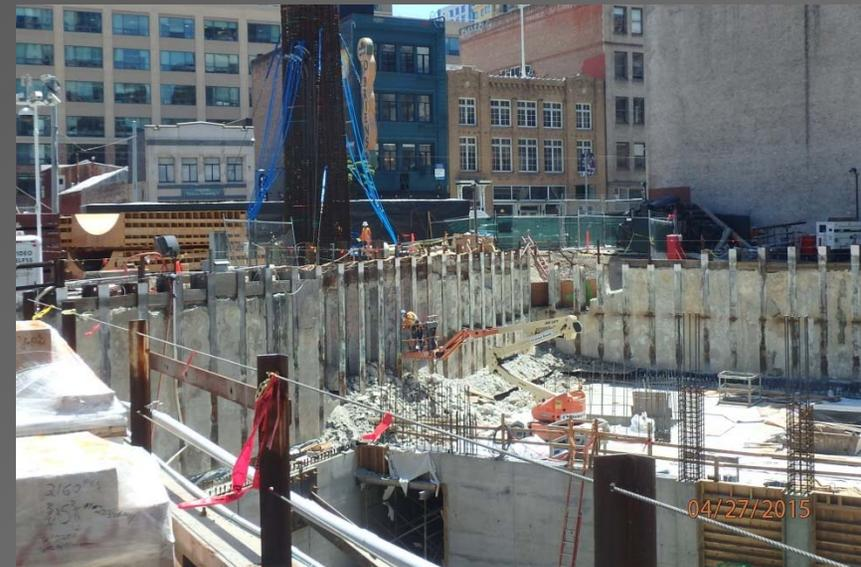
Below Right: Removal of shoring wall to allow for vehicle ramp tie-in.
