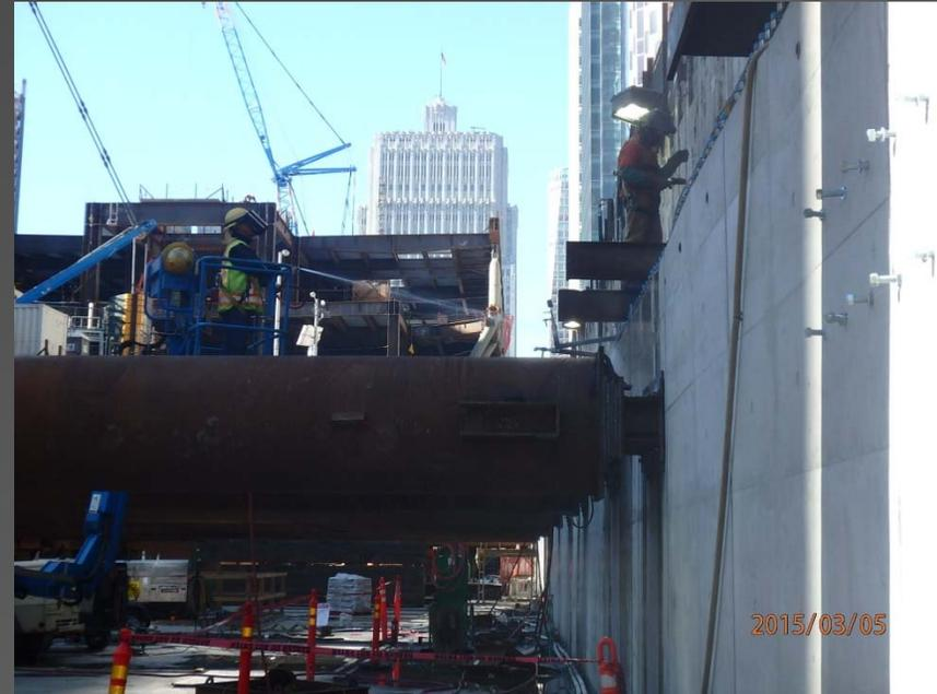
Above Right: RA level bracing at 3<sup>rd</sup> lift walls.
