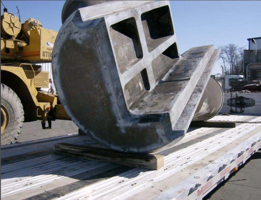
Above and Right: One of the largest cast nodes (approximately 20 tons) prepared for transit to the steel fabricators in Oregon. Eventually will be installed at the east end of the project along Beale Street.
