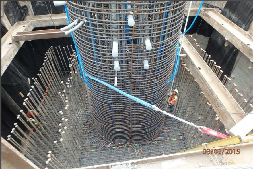
Above: Pylon 9 pile cap and start of reinforcing steel.
