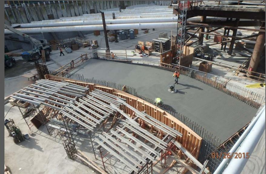
Above and Below Right: Concrete placement and continuing formwork and reinforcing steel for bike and vehicle ramp from street level to lower concourse.
