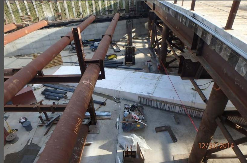
Above Left: West end train platform level with lower concourse formwork removed.
