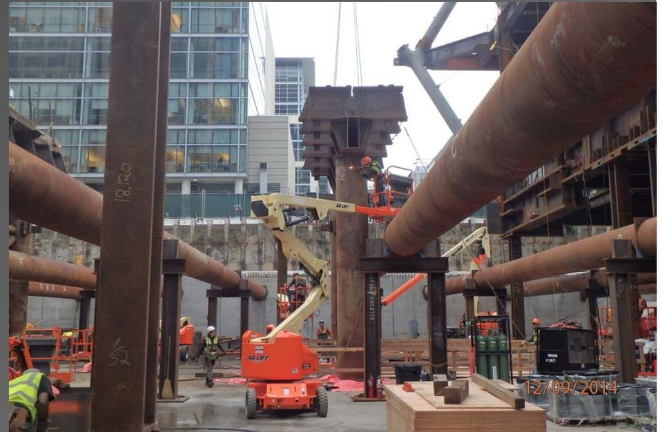
Above and Right: Removal of next section of access trestle for continuation of steel erection.
