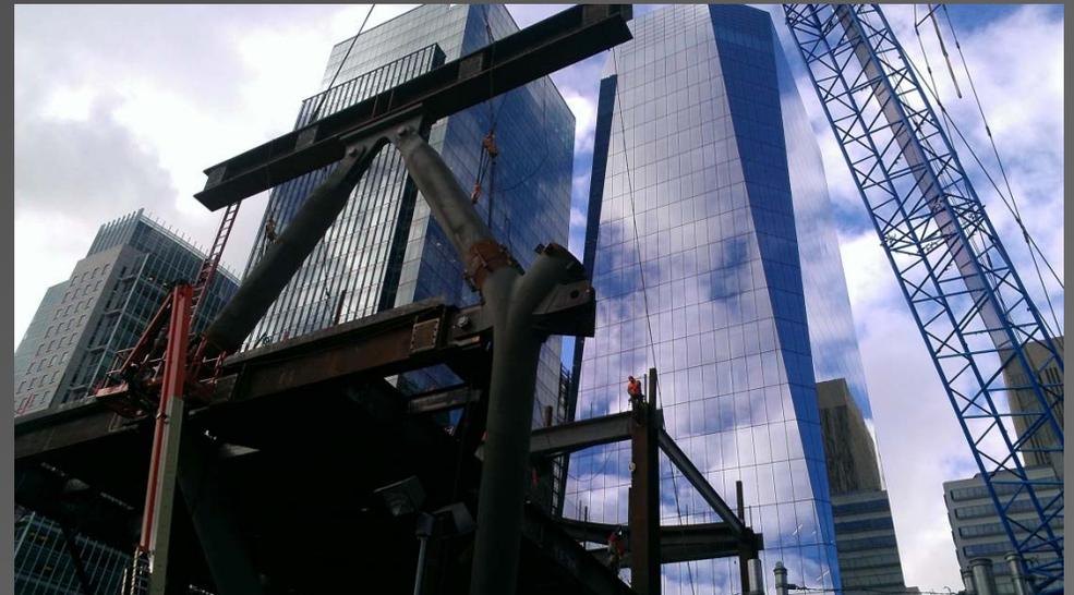
Above: Cast nodes and pipe columns connecting bus deck and roof park.
