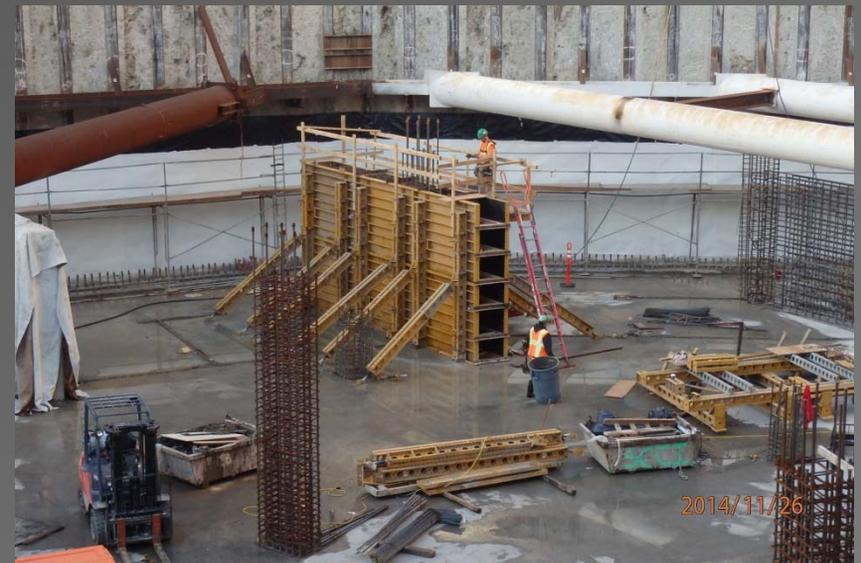
Below Right: West end lower concourse level interior walls and waterproofing ready for 3<sup>rd</sup> lift walls.
