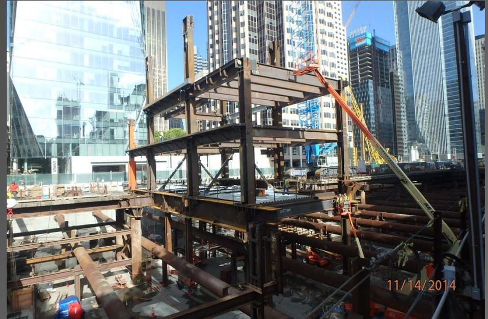
Above: Ground, mezzanine and bus deck level steel erected.
