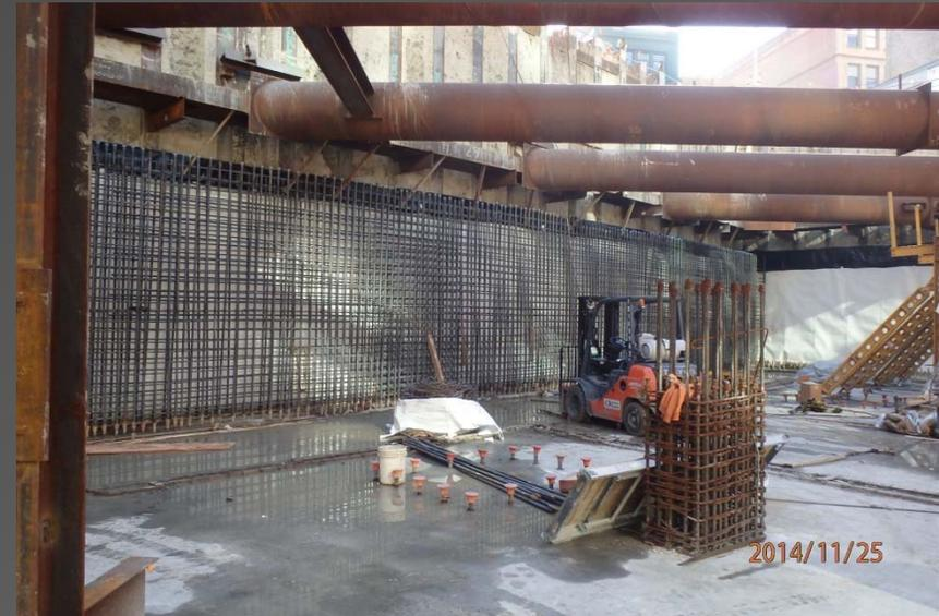
Above Right: Southwest end, reinforcing for 3<sup>rd</sup> lift walls.
