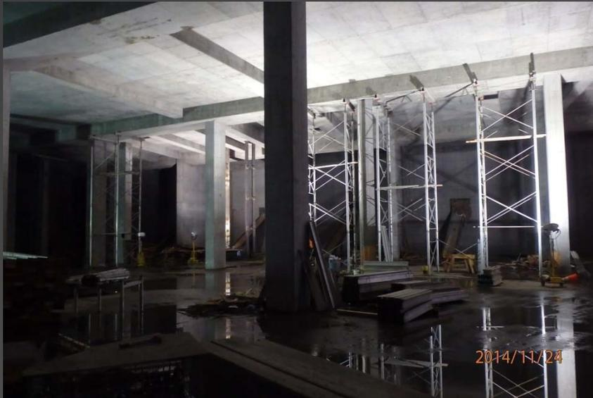
Above Left: West end train level, lower concourse formwork being removed.
