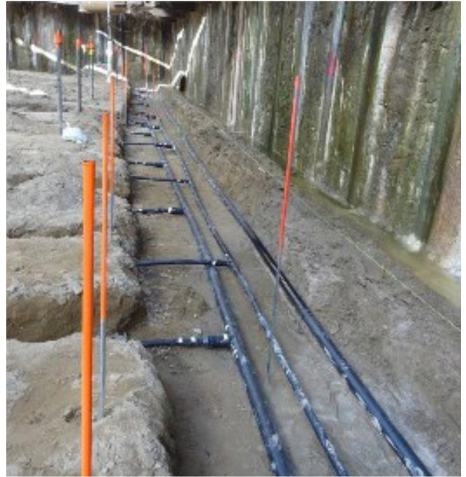
Geothermal piping under the foundation of the Transit Center will reduce heating and cooling needs for the Transit Center, helping to achieve a LEED Gold rating.
