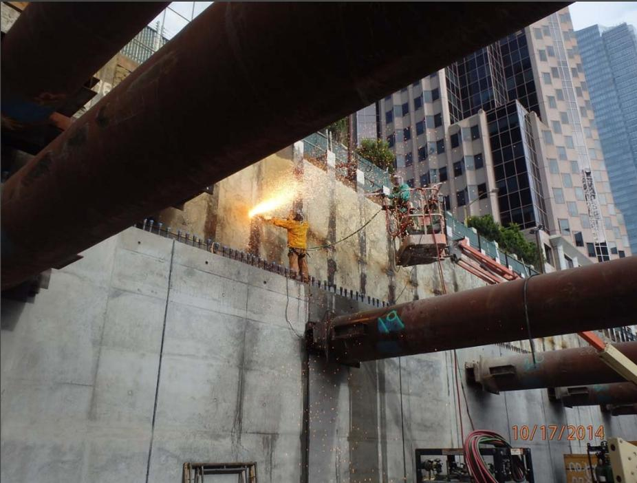
Above: Removing all Bracing Level A supports.
