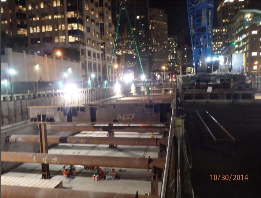
Left: Transfer Girder hoisted into place.
