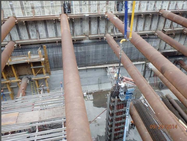
Above Left: Wall lift 1 reinforcing steel installation.
