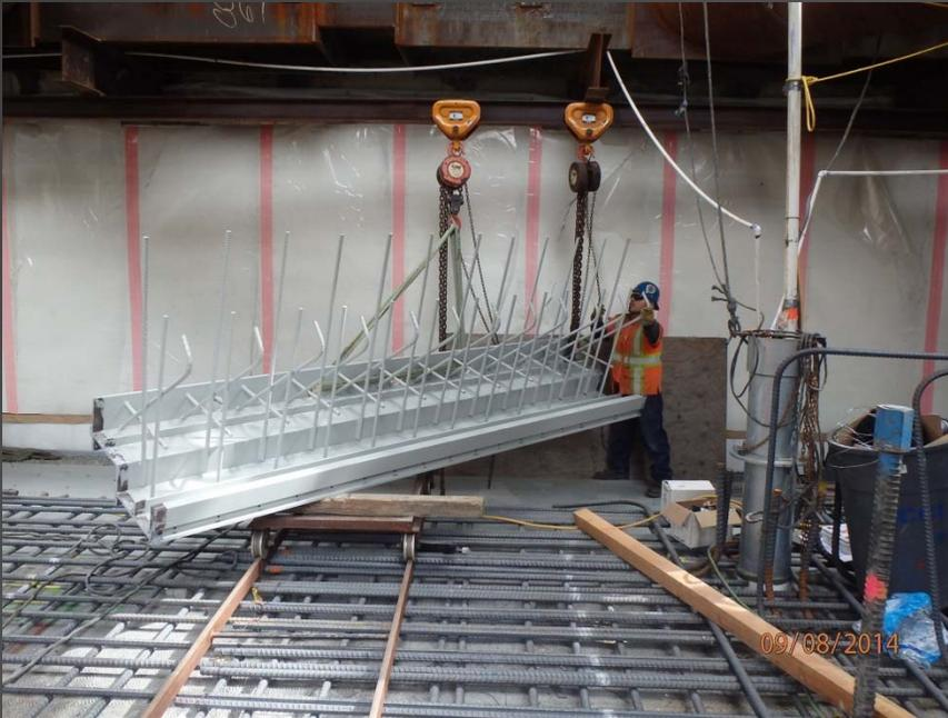
Above: Positioning seismic joint, note rail system.
