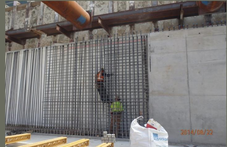
Completion of 80% of the central zone lower concourse level slab has allowed for the placement of 3<sup>rd</sup> lift foundation walls and re-bracing. These are the items that need to be completed prior to start of structural steel.
