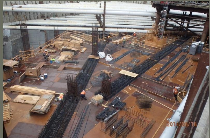
Primary focus in the western zone has been the completion of the Lower Concourse level decking for concrete placement.
