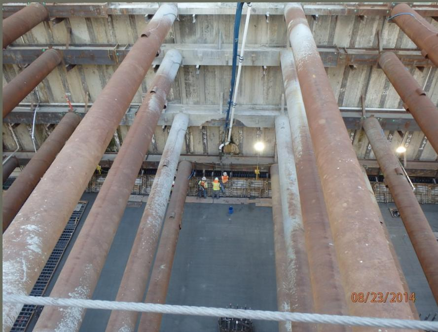
Mat foundation slab placement #15, reinforcing steel for mat foundation pour #16 (the last one).
