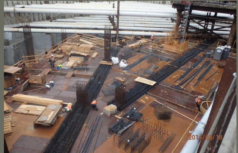
Primary focus in the western zone has been the completion of the Lower Concourse level decking for concrete placement.
