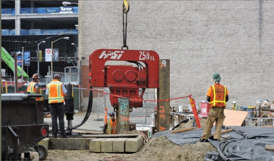
Installation of shoring at Pylon 9 location in preparation for Barrette Pile installation work has been completed. Cable-stayed pylon structure requires the specialized *barrette pile* foundation to accommodate lateral seismic forces without impacting train box.
