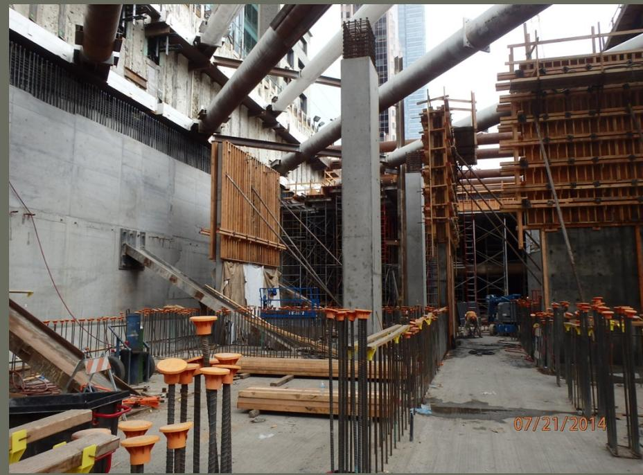
Completion of perimeter lift 2 walls and internal concrete walls prior to start of Lower Concourse decking.
