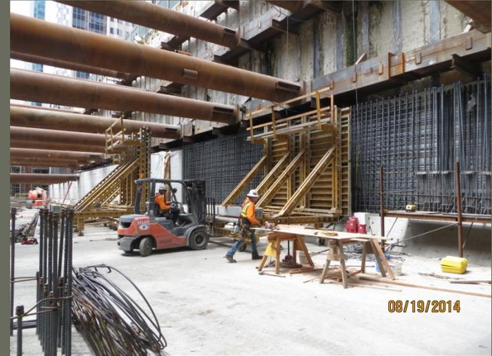
Eastern zone bracing removal, 1<sup>st</sup> and 2<sup>nd</sup> lift wall construction.
