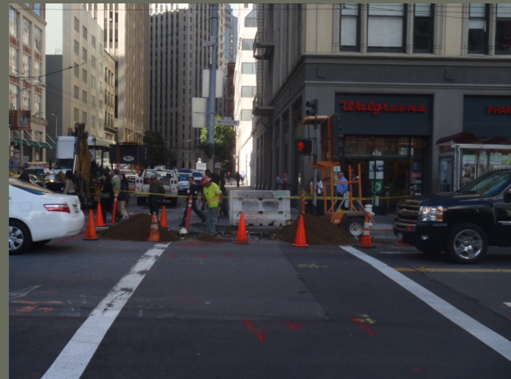
Potholing for AWSS on Mission Street
