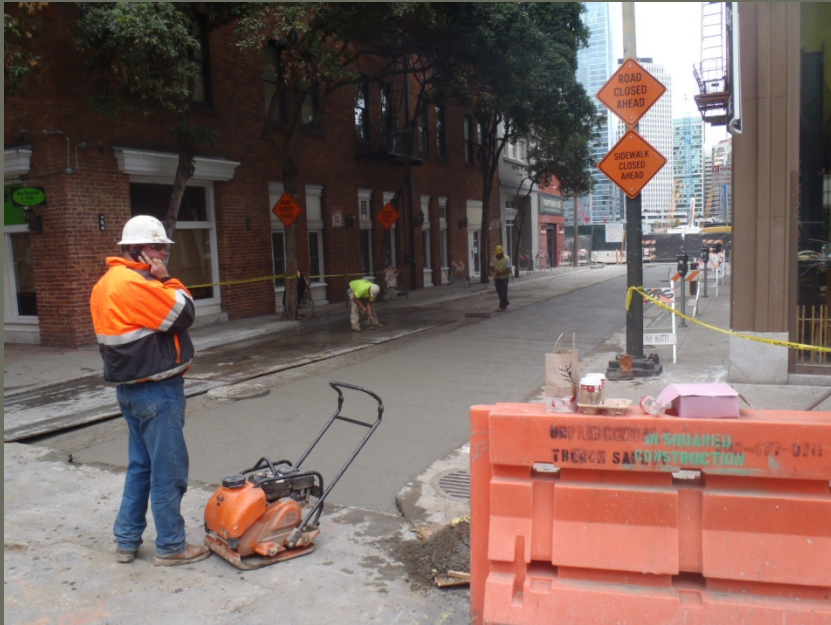
Restoration of Natoma St. at 2 nd Street
