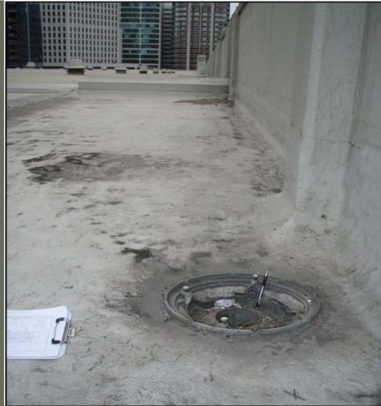
Transbay Terminal Roof - Asbestos Coating on Parapet
