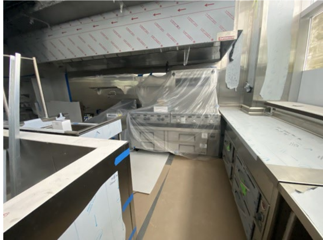
Tycoon Kitchen – equipment being installed
