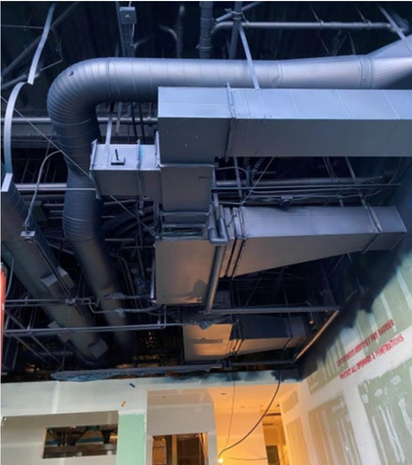
Per Diem – newly painted ceiling
