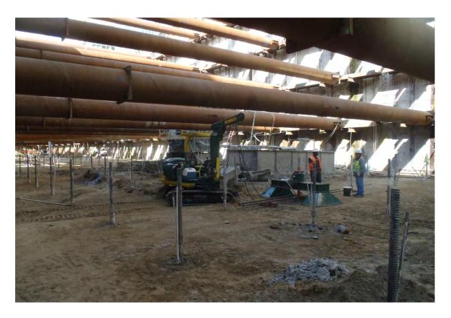
Micropile Pull Test Underway
