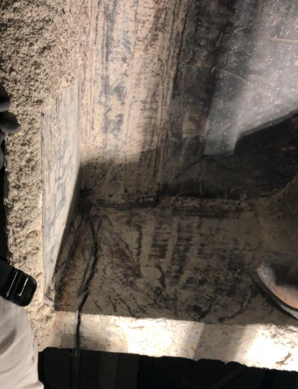
fissure located on flange on the bottom portion of the beam that spans over Fremont Street. (fireproofing removed to identify extent of fissure)
