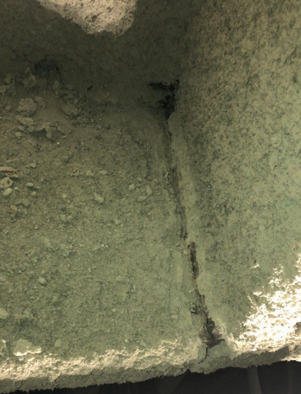
fissure located on flange on the bottom portion of the beam that spans over Fremont Street. (fireproofing intact)
