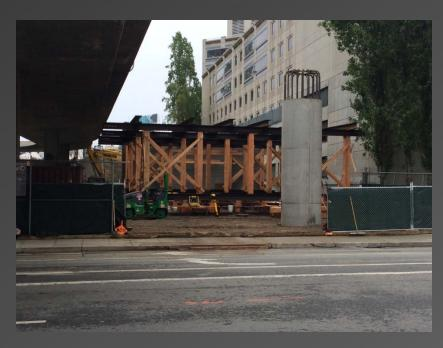
Above Left and Right: Falsework erection in progress, southside of Folsom Street.
