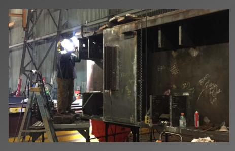
Above: Pipe column fabrication at Oregon Iron Works (OIW).
