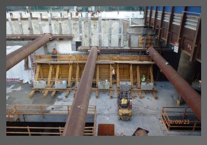
Above: RA Level bracing in place and A Level bracing and waler removed.
