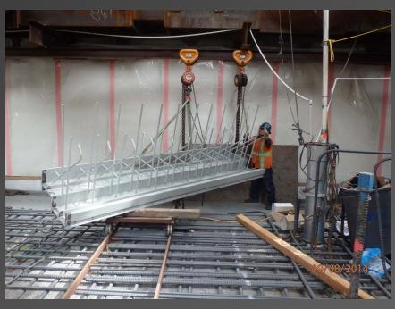
Above: Positioning seismic joint, note rail system.
