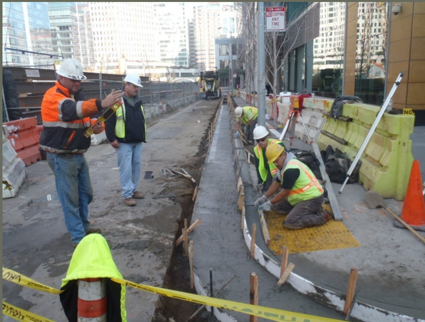
Restoration of Natoma St. behind 400 Howard Street
