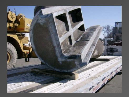
Above and Right: One of the largest cast nodes (approximately 20 tons) prepared for transit to the steel fabricators in Oregon. Eventually will be installed at the east end of the project along Beale Street.
