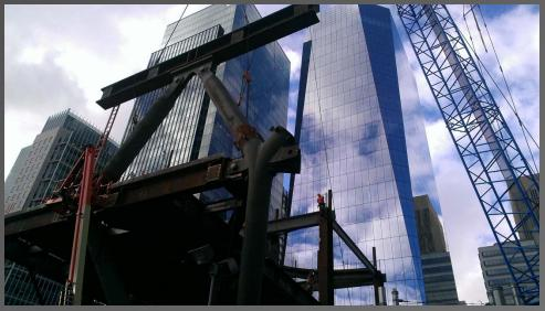
Above: Cast nodes and pipe columns connecting bus deck and roof park.
