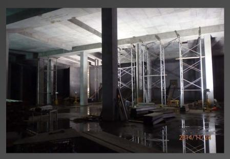
Above Left: West end train level, lower concourse formwork being removed.
