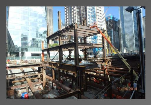
Above: Ground, mezzanine and bus deck level steel erected.
